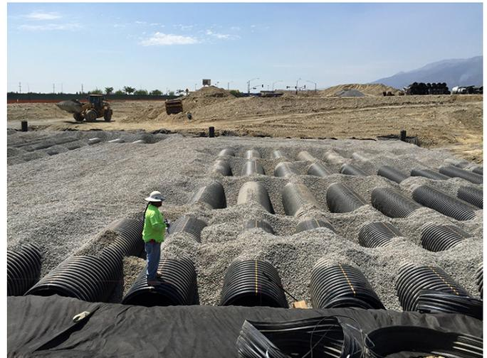
HDPE was selected over other pipe material alternatives for this job according to Currence. "We were told that the engineer typically considers both corrugated metal pipe and corrugated HDPE pipe for these types of projects, but prefers to use HDPE when there is no significant difference in price. He feels that HDPE pipe offers greater longevity."
